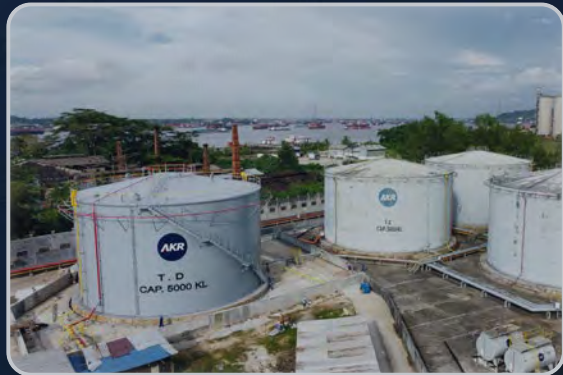
Construction Storage Tank 5.000 KL & Supporting Facilities
