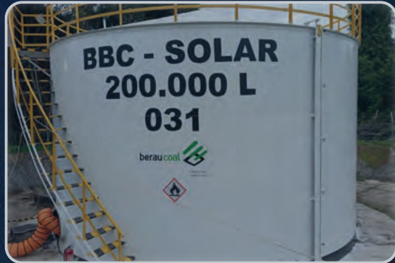
Repair and Improvement Storage Tank 1×200 KL
