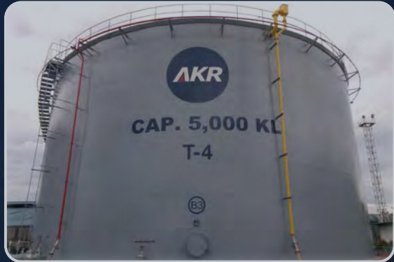
Repair and Improvement Storage Tank 1×5.000 KL
