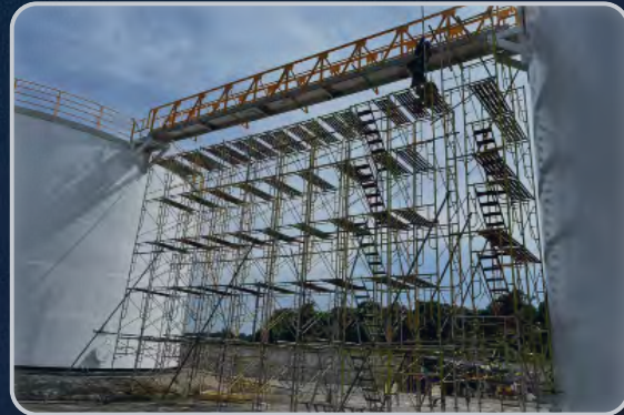
Repair and Improvement Storage Tank 2x2000 KL
