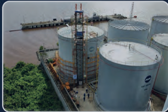
Repair and Improvement Storage Tank 1×3.500 KL
