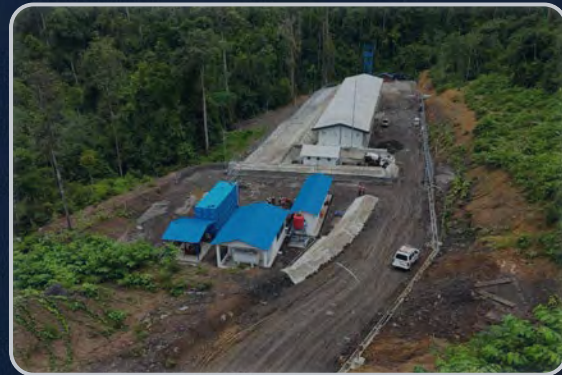
Magazine Warehouse Construction
