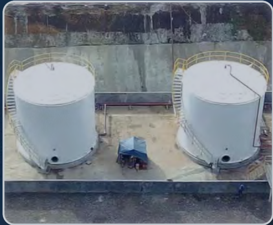
Construction 2×250 KL Storage Tank
