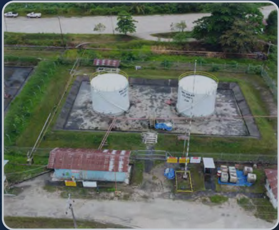
Repair and Improvement Storage Tank 2×250 KL
